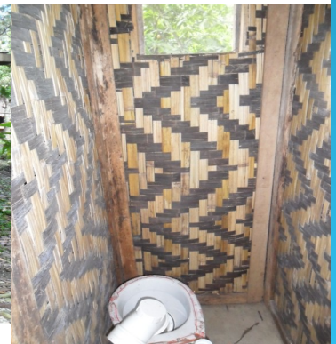
One of the two toilet rooms.
