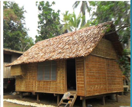
Ando Local Church guest house and hall.
